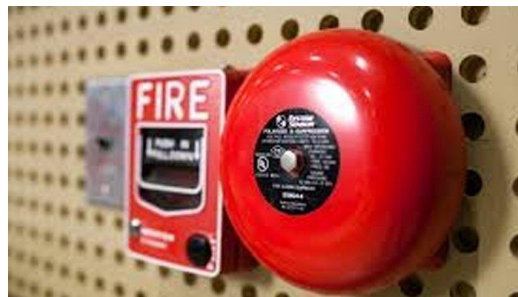
Gambar 2. 3 Alarm kebakaran Sumber : (Yudhi, 2018)
