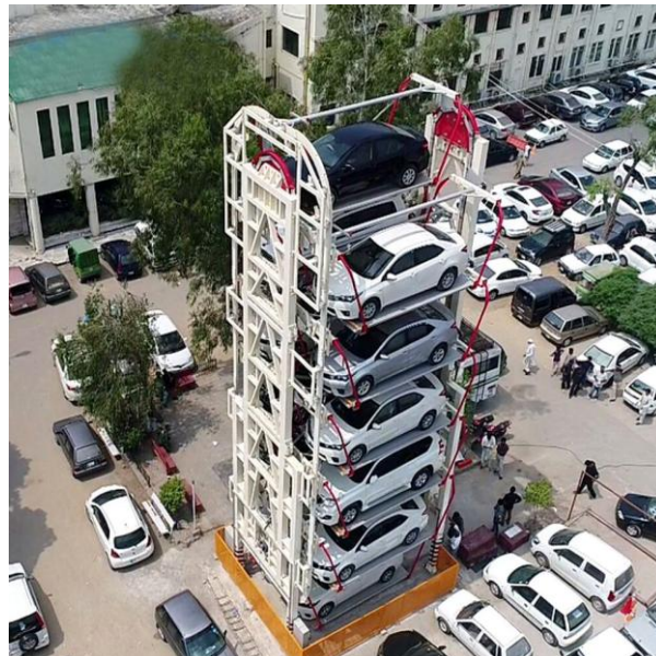
Gambar 2. 1 Mekanisme Rotary Parking vertikal [22]
