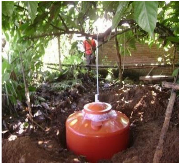
Gambar 0.5 Digester tipe fixed dome
