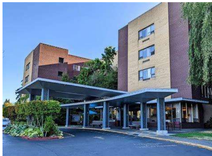
Gambar 2.14 Tampak Providence Mount St. Vincent
