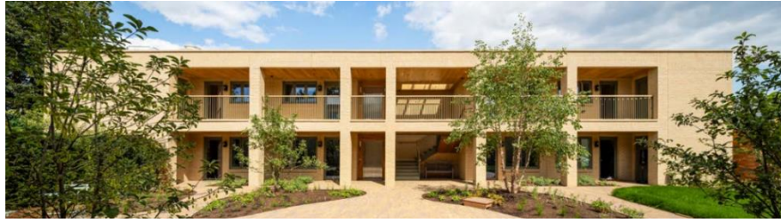
Gambar 2. 53 Gedung Residensial Hope Street
