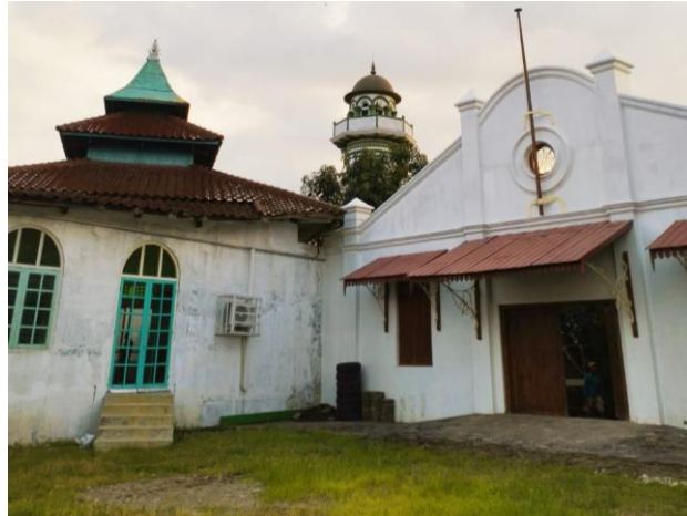
Figure 4.1 Documentation of Physical and Architectural Observations of the Masjid Menara Layur
