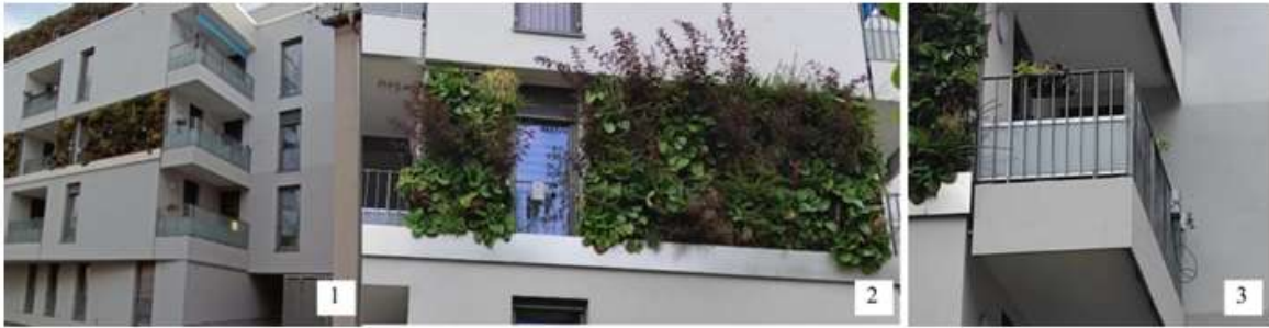
Gambar 2.6 GreenONE Residential Building , Nordhausen, Jerman
