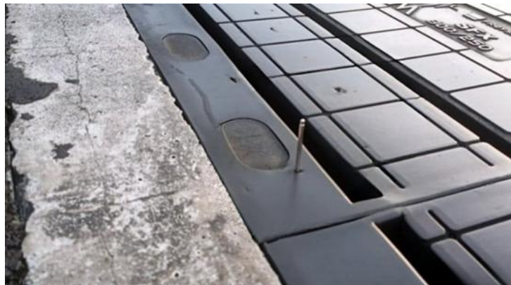
Figure 1. Foreign Object in MBZ Expansion Joint
