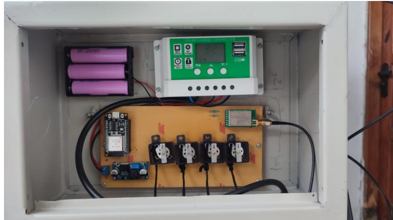
Gambar 4. 6 Hasil Perakitan panel Box Transmitter
