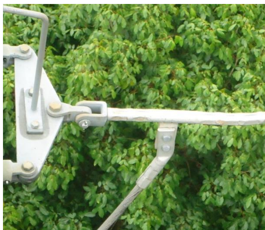
Gambar 2.23 Jumper Joint
