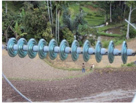
Gambar 2.26 Insulator gelas / kaca
