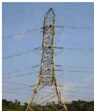
Gambar 2.5 Lattice Tower
