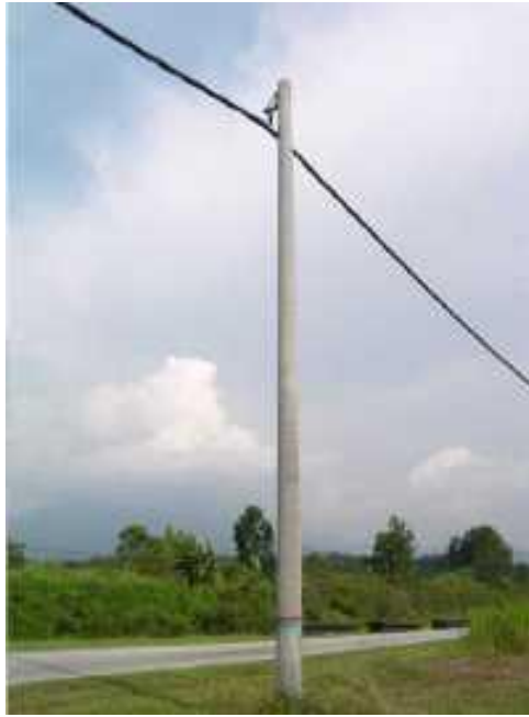
Gambar 2.7 Concrete Pole Tower
