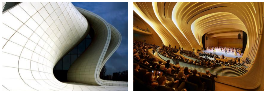
Gambar 2.40. Eksterior dan Interior Hayder Aliyev Center, Azerbaijan Sumber : https://www.archdaily.com/
