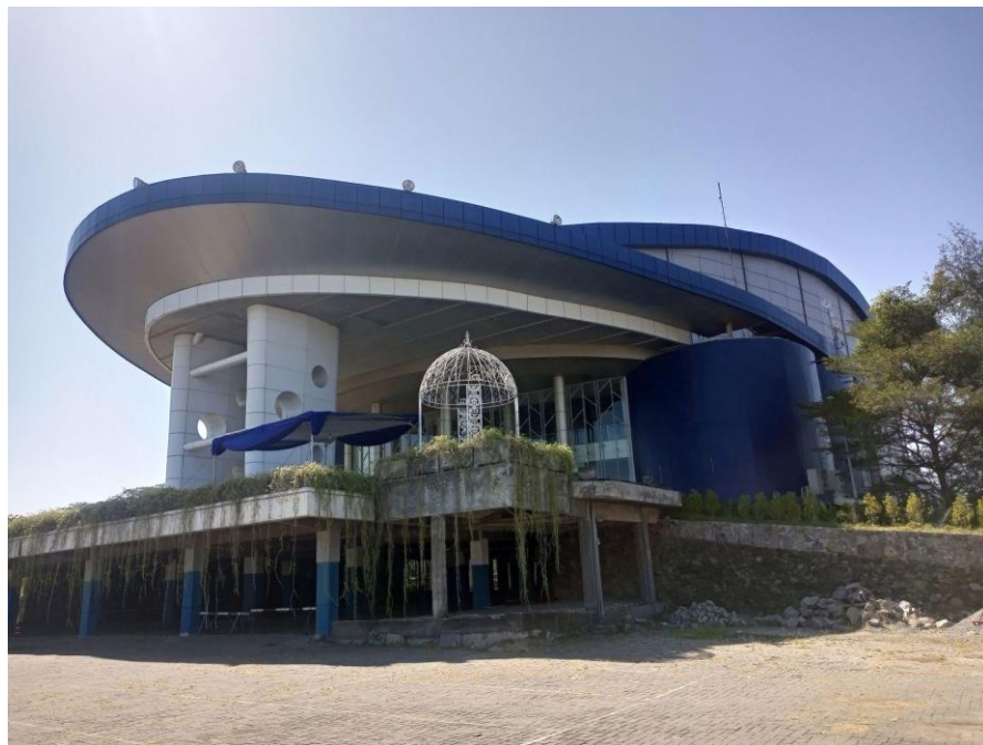
Gambar 2. 2 Tampak Samping MCC
