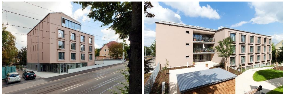
Gambar 2. 15 Veronica House Elderly Care Facility
