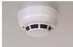
Gambar 4. 14. Smoke Detector
