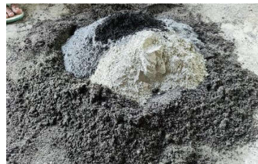
Gambar 3. 28 Mencampur Bahan Material Paving Block
