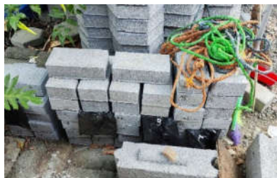
Gambar 3. 32 Curing Paving Block
