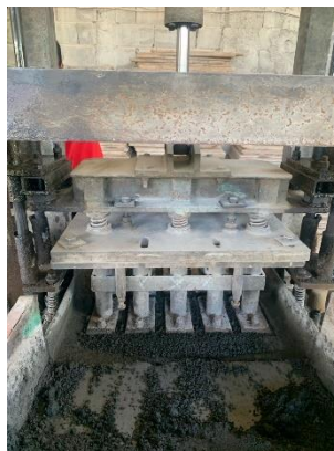
Gambar 3. 36 Proses pencetakan paving block
