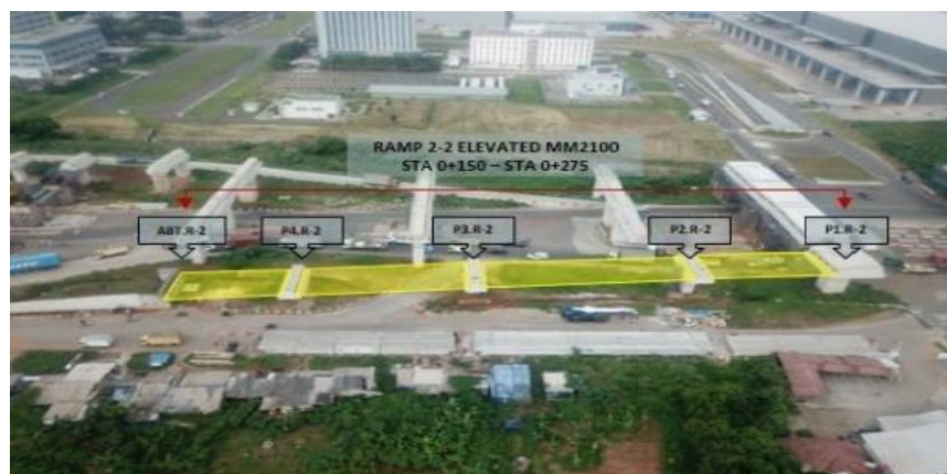
Gambar 3.2 Ramp 2.2 Elevated MM2100
