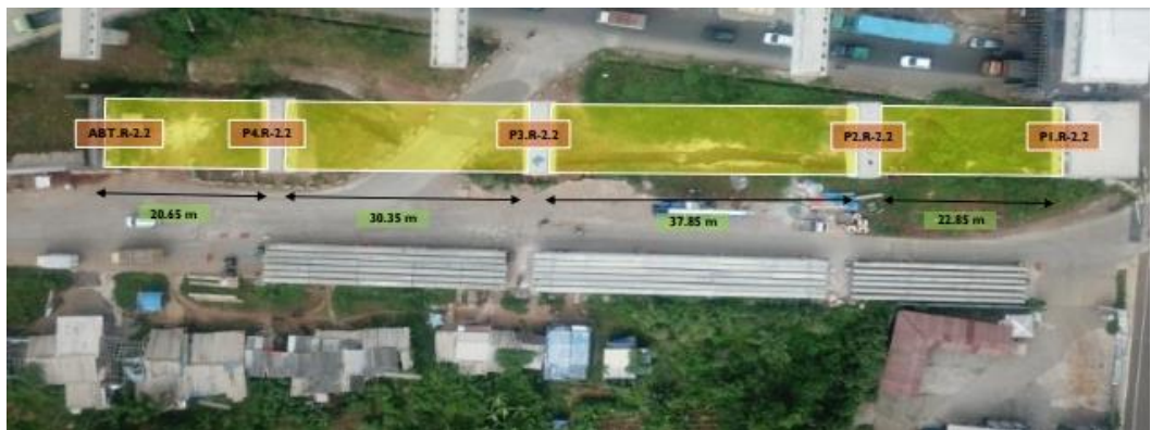
Gambar 3.1 Ramp 2.2 Elevated MM2100
