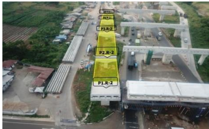
Gambar 3.3 Ramp 2.2 Elevated MM2100
