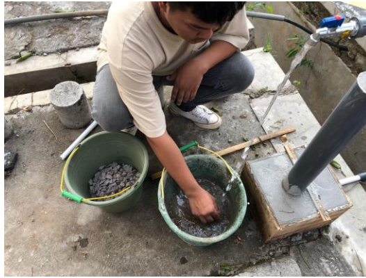
Gambar 3.6 Pencucian Agregat Kasar
