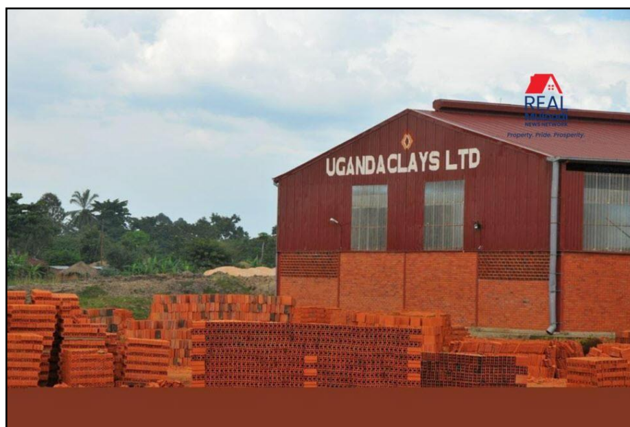
Figure 2.1 Uganda Clays LTD Head Quarters in Kajjansi
