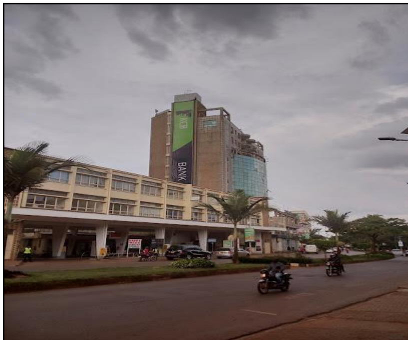
Figure 2.15 Kenya Commercial Bank Ltd
