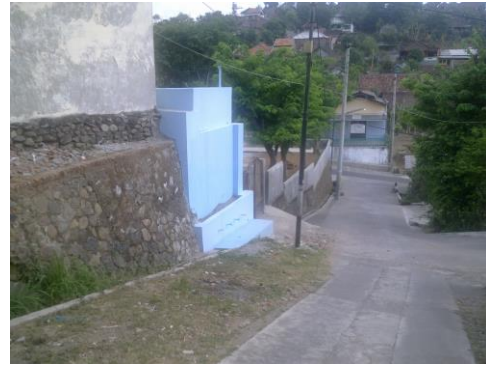
Figure 7. Completed Storage A with Water Taps Outside.
