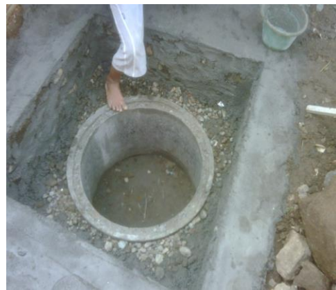
Figure 3. Small Recharge Well Made Underneath the Barrels.
