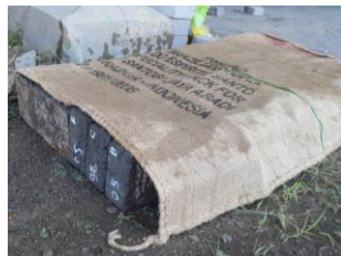
Gambar 3. 47 Curing paving block
