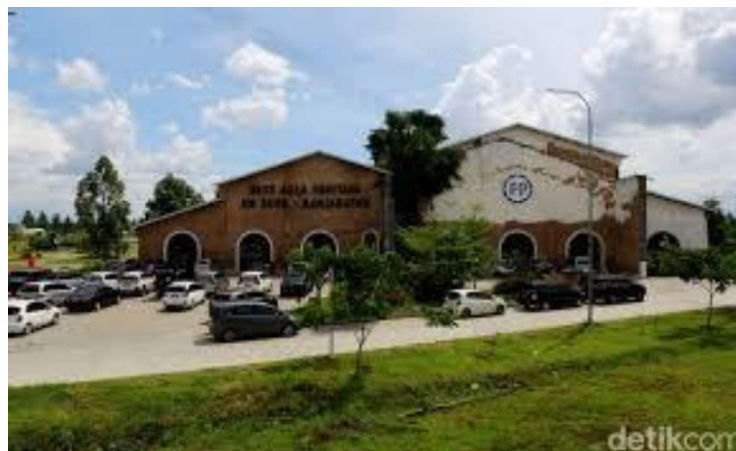
Gambar 2.11 Rest Area KM260B
