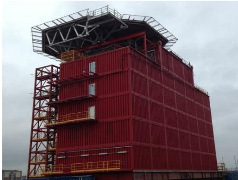
Figure 14. Platform AUK – North Sea
