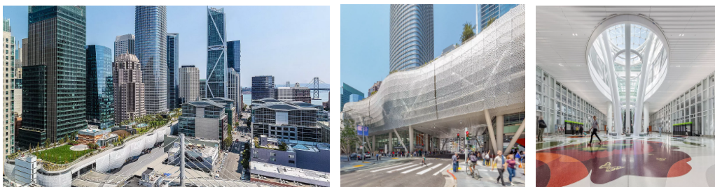
Gambar 2.10 Salesforce Transit Center Sumber: https://ww3.rics.org/uk
