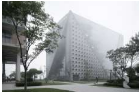
Gambar 32. Tampilan Fasad 1 (Sumber: Atelier Alter Architects)
