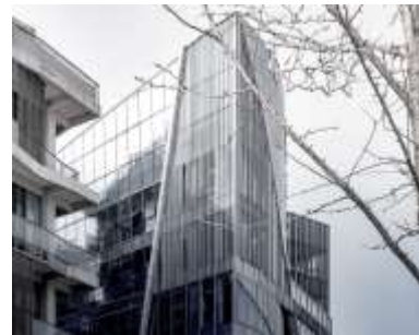
Gambar 33. Tampilan Fasad 2 (Sumber: Atelier Alter Architects)
