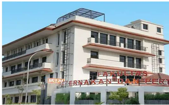
Gambar 3.4 Gerbang Gedung Dekanat FPP Undip
