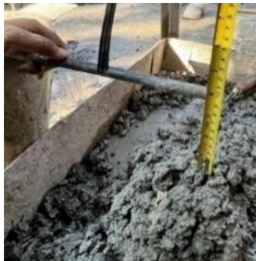
Gambar 4.2. Hasil Uji Slump Beton Normal
