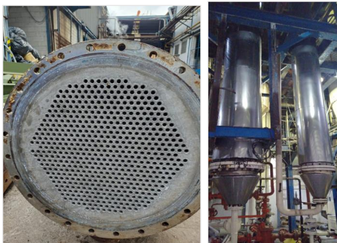
Gambar 2. 6 Heat Exchanger
