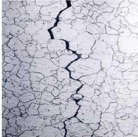
Gambar 2. 6 Stress Corrosion Cracking (Sumber: AMPP – Stress Corrosion Cracking, ampp.org )
