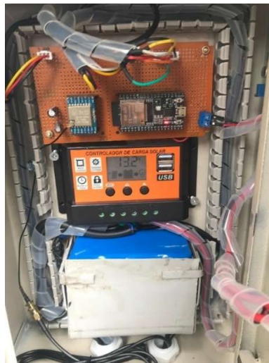
Gambar 4. 20 Hasil Perakitan Panel Box Transmitter
