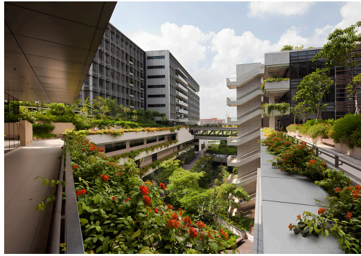
Gambar 2.37 Khoo Teck Puat Hospital Facade
