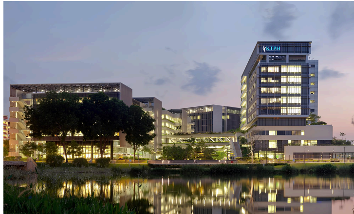
Gambar 2.36 Khoo Teck Puat Hospital Facade
