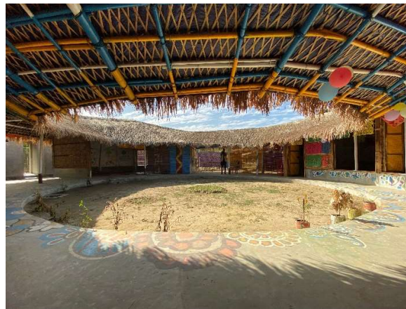
Gambar 2.5 Beyond Survival Comunity Center for Women 2 Sumber Archello
