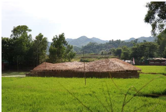
Gambar 2.7 Beyond Survival Comunity Center for Women 4 Sumber Archello
