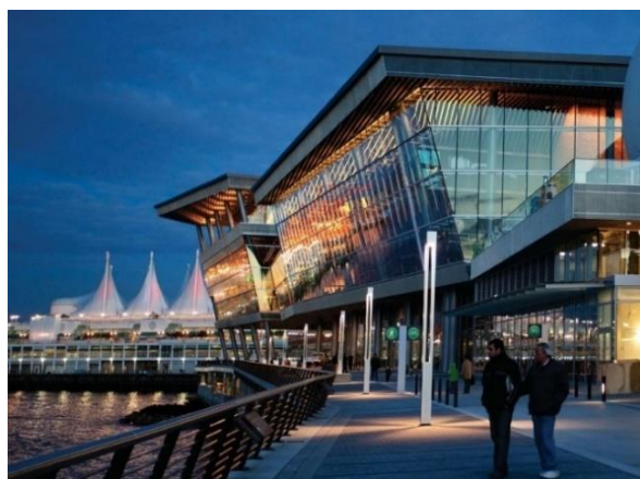
Gambar 15 .Vancouver Convention Centre West
