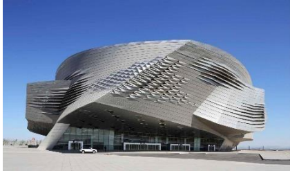
Gambar II.31 Dalian International Conference Centre di China
