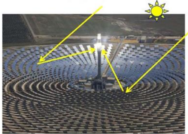
Gambar 2. 5 Sistem CSP tipe Central Receiver Tower
