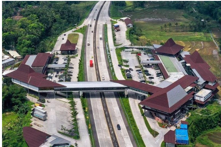
Gambar 2. 5 Rest Area KM 456 Sumber: www.mbtech.info
