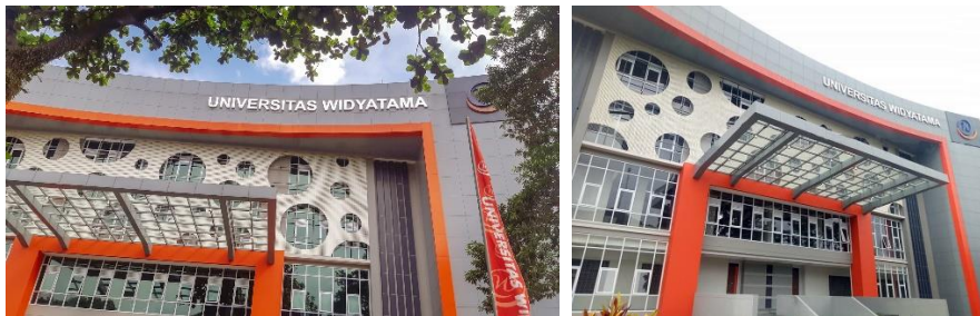
Gambar 2. 19 Gedung PKM Universitas Widyatama (Sumber : www.widyatama.ac.id )
