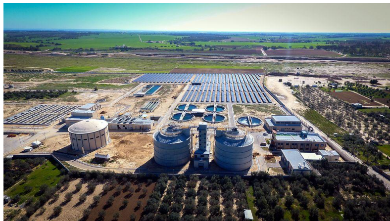
Gambar 2.2 Project Example: Gaza Central Wastewater Treatment Plant
