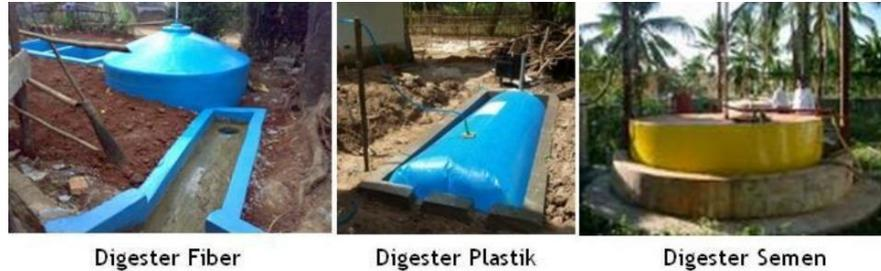
**Gambar 2. 2.** Contoh digester anaerobic (Waskito, D., 2011)
