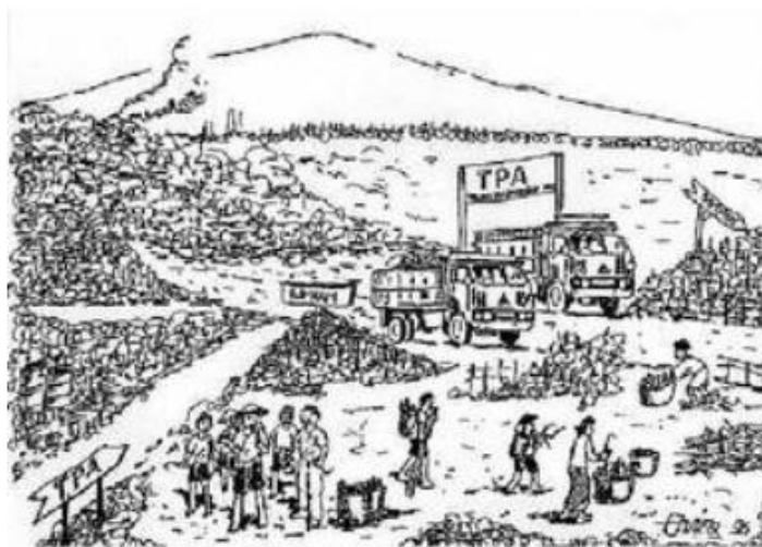
Gambar 2.2 Open dumping landfill
